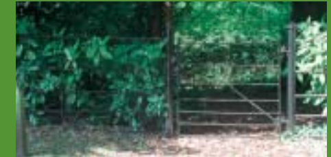
Iron gate and matching railings – The Old Rectory.
